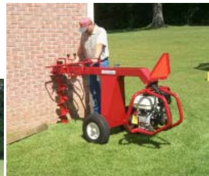
Figure 11B Up-close Drilling
